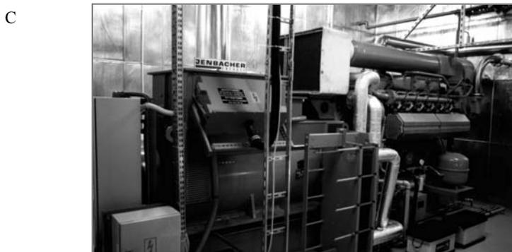
Fig. 3. Absorption heat pump (Sanyo, 2.7 MW) cooperating with high-temperature boiler (Viessmann, 1.9 MW) in Mszczonów geothermal plant (A). Peak-load boiler house in Zakopane (B). Co-generator unit (Jenbacher, 0.54 Mw<sub>e</sub> + 0.7 Mw<sub>t</sub>) in boiler house in Zakopane (C)
